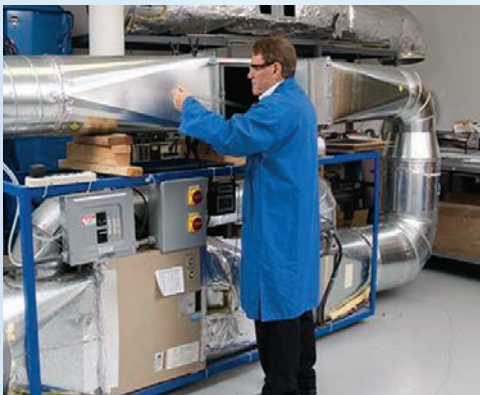
HVAC Duct System for Product Testing
